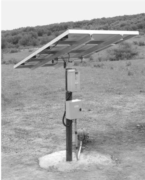
Setting an array pole in concrete.
