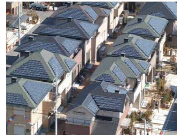
building integrated PV
