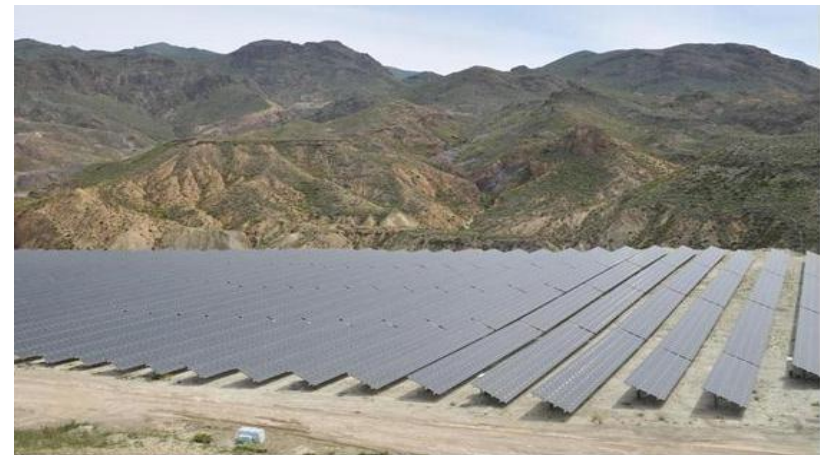
Megawatt Power Plant, Spain
