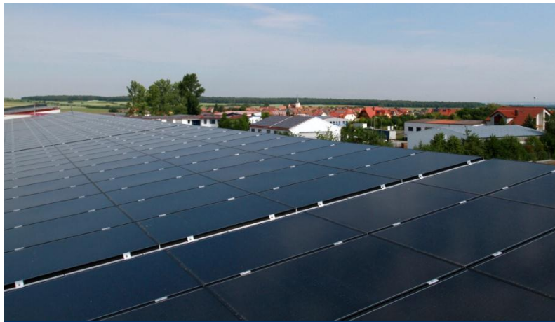
Parking Lot Rooftop, (from above) Germany
