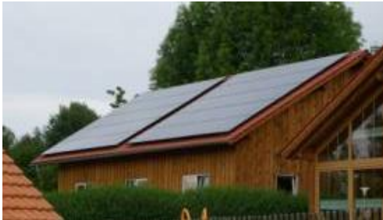
Residential Rooftop, Germany
