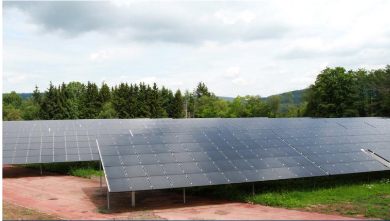
Power Plant, Germany
