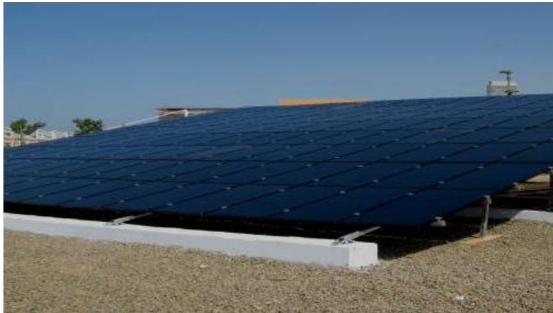
Microgrid, Saudi Arabia
