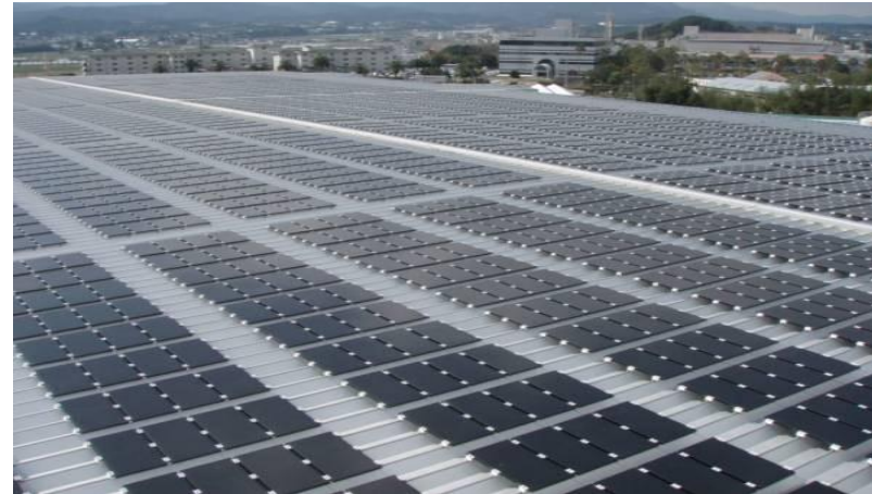
Commercial Rooftop, Japan
