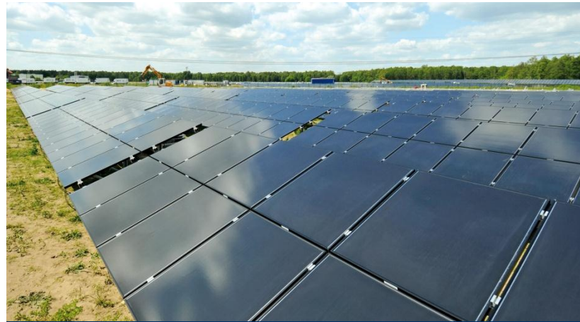
Megawatt Power Plant, Germany
