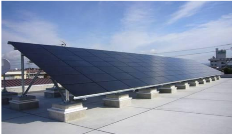
Commercial Rooftop, Japan
