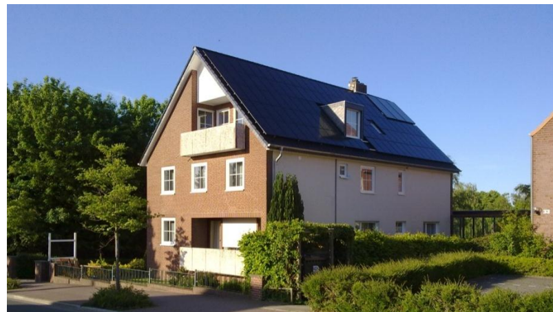
Residential Rooftop, Germany
