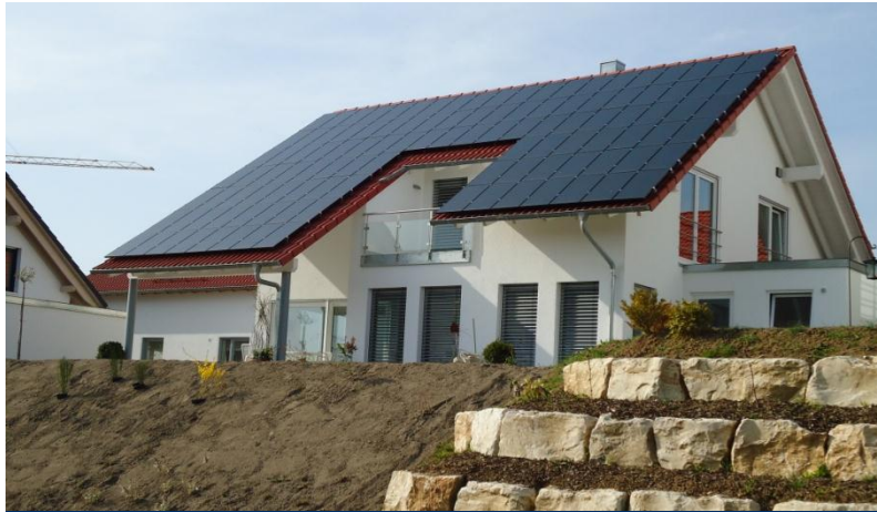
Residential Rooftop, Germany
