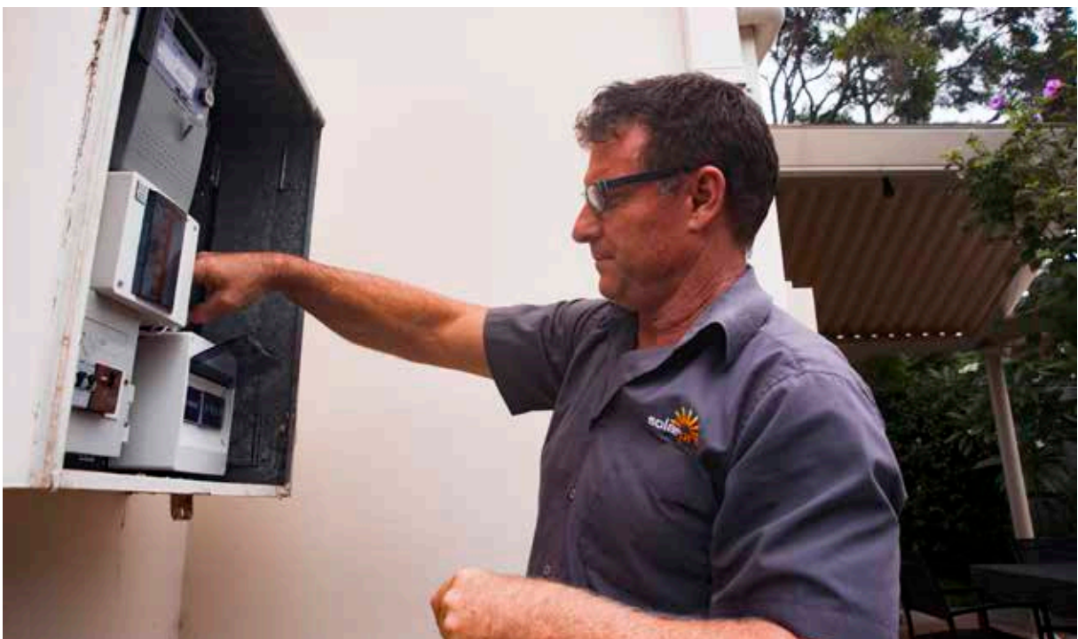
Photo courtesy Reposit Power
