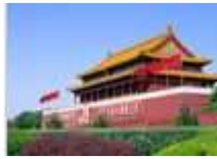
Tian An Men Square Project
