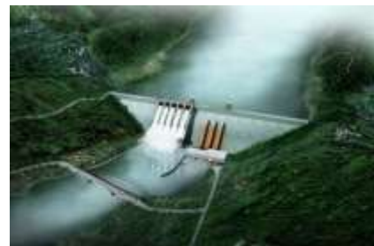
Vietnam Hydro Power Plant
