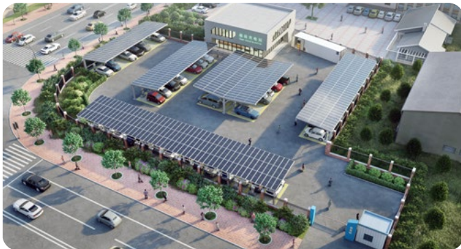
PV Charging Carport With Storage
